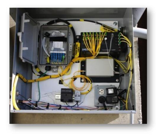
The control panel containing Luna's sensing instrumentation is located more than 1.5 miles from the bridge in a more controlled environment allowing for easier access. A fiber optic trunk line that was already in place is used to connect instrumentation with sensors installed on the bridge.
